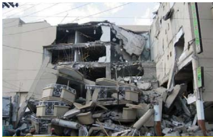
Damages caused by the October 8, 2005 quake in Pakistan
