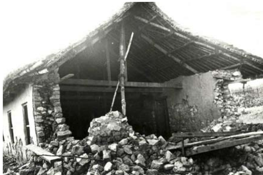
Damage caused by the 1988 Earthquake, Dharan
