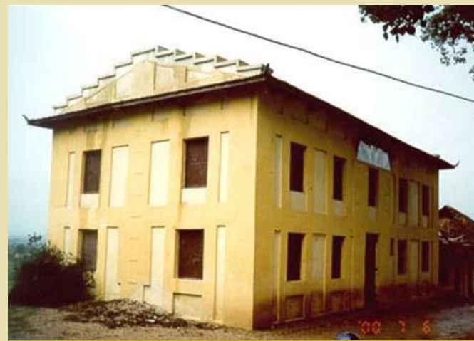
Bhubaneshori Lower Secondary School- After
