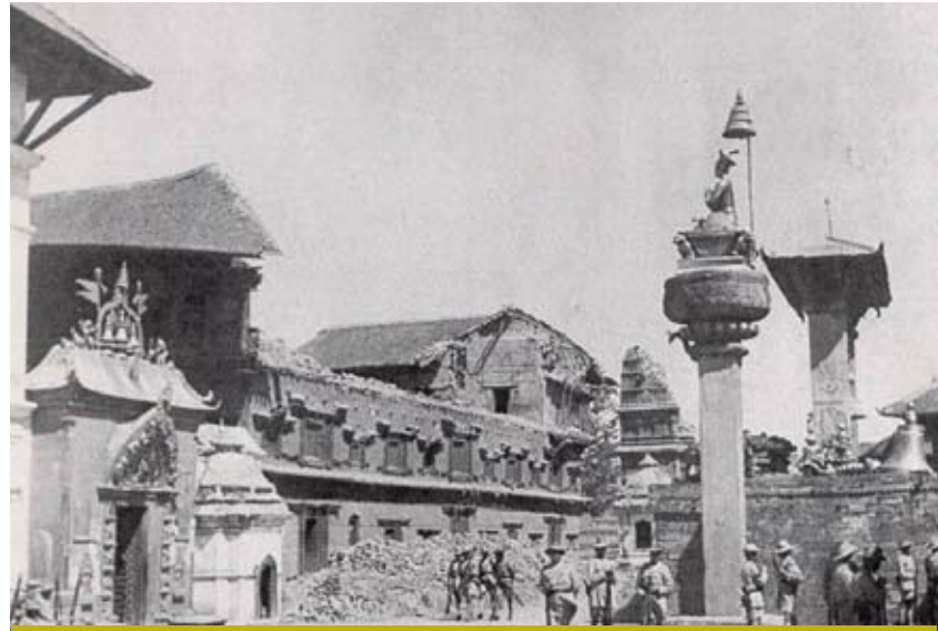
Damage caused by the 1934 Earthquake, Kathmandu
